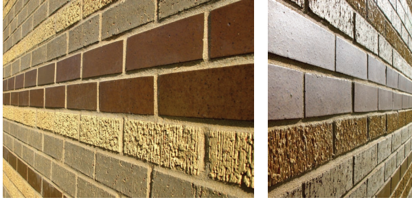
The same brick when viewed from different angle relative to the sun. Smooth goes from dark to light, textured goes from light to dark
