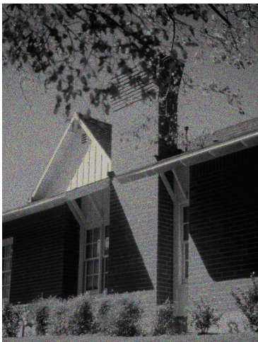
Overhangs which protect windows from harsh sunlight and add visual interest to the facade.
